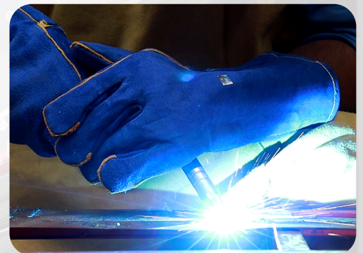
Example for welding using AUTO MIG Machines
